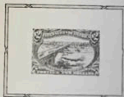
Mississippi River Bridge
